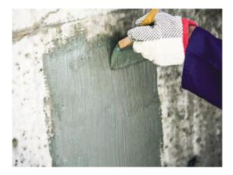
While the substrate is damp but free from standing water, apply the mixed product a minimum of 2 coats by medium hard short bristle brush, trowel or roller checking that the first coat is at a minimum wet film thickness of no more than 1.5mm and no less than 0.5mm. The product should always be finished in one direction.
